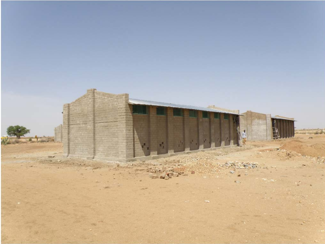
Permanent classrooms for a school in Nyala
