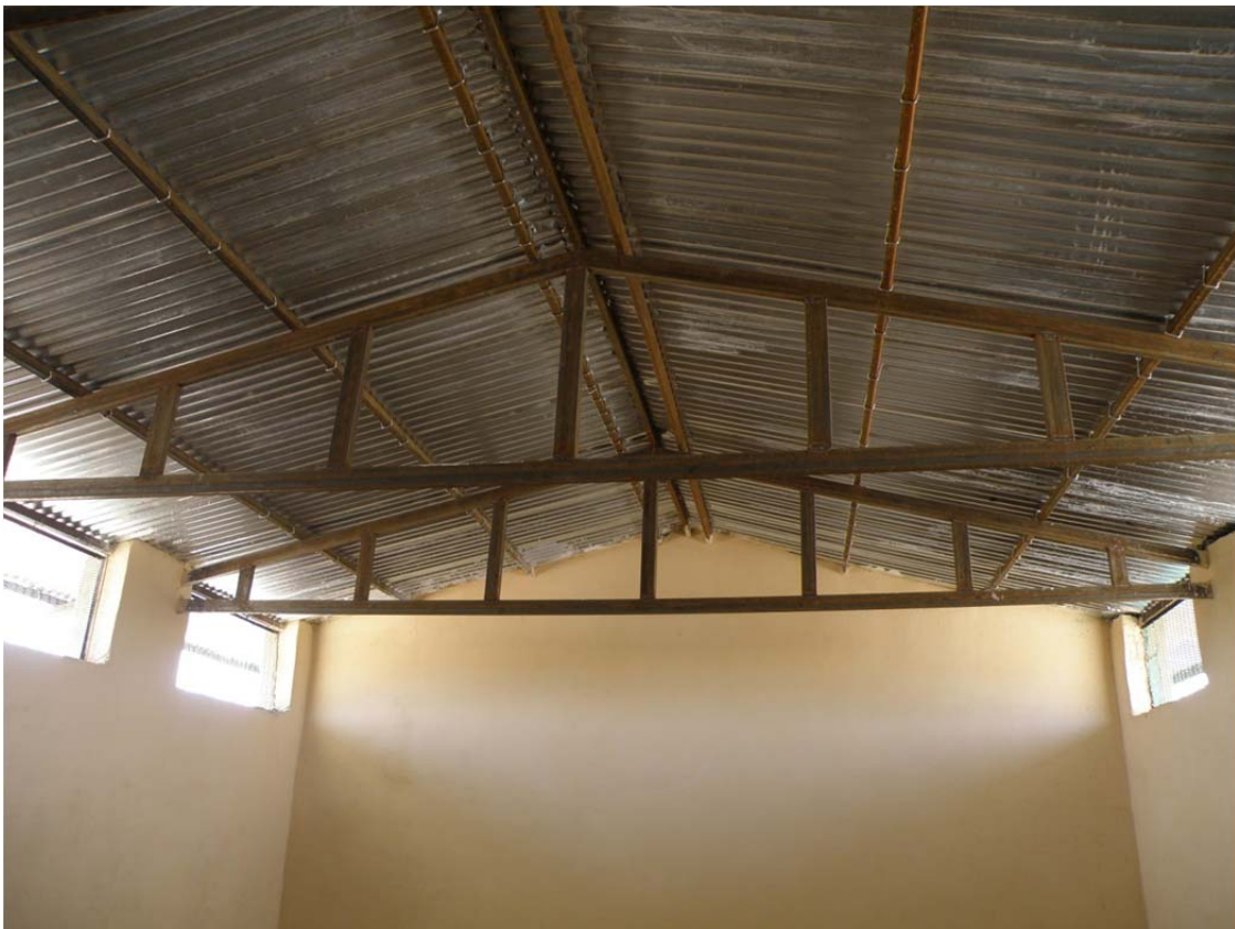
Inside view of a permanent classroom
